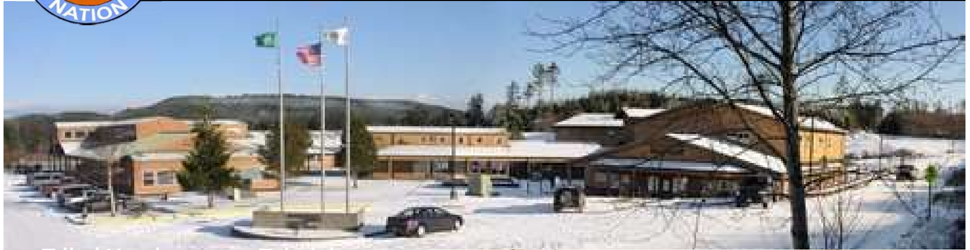
Tribal Headquarters, Taholah
